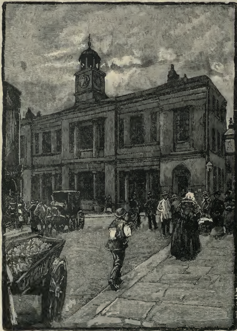
THE OLD TOWN HALL, CROYDON, BEFORE DEMOLITION. (See page 176.)
